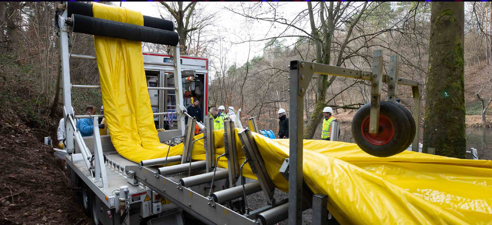
IMPREG liner being installed on various sites.
